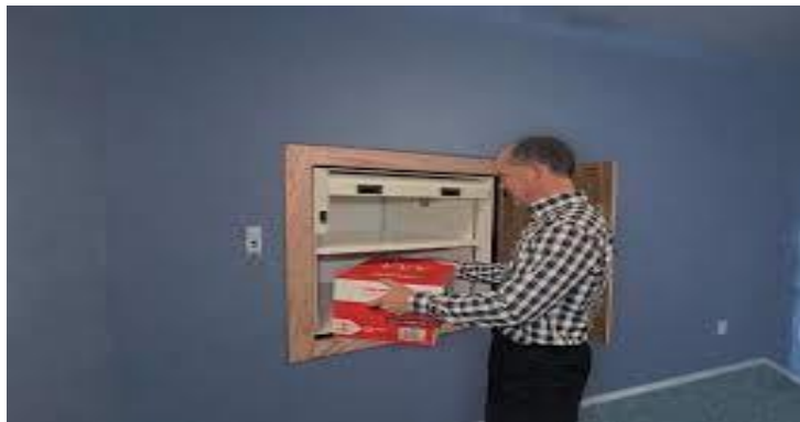
Gambar 5.16 Dumb Waiter elevators rekam medis
